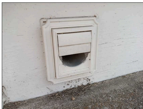
Missing dryer vent louver
