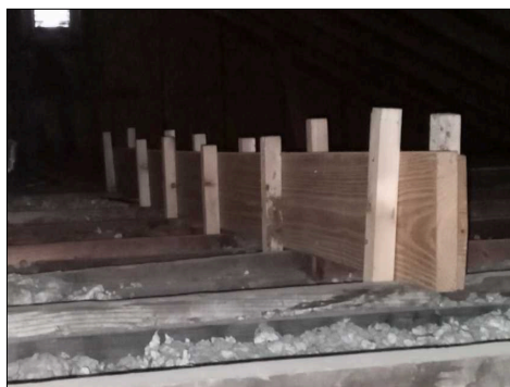
Load bearing wall support header is missing joist hangars
