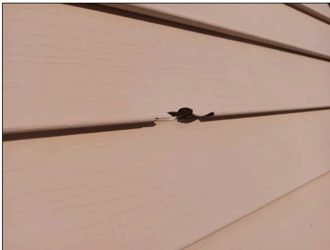
Holes in the exterior siding
