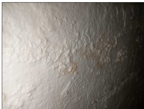
There is some moisture staining and scaling to the foundation visible from the basement
