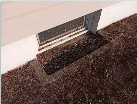
The basement window wells may need window well covers installed
