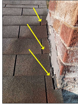
Gap where the chimney meets the roof
