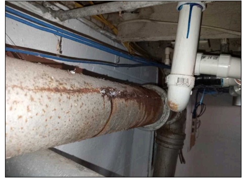
The cast iron sewer drain pipe is cracked
