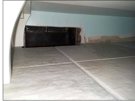
A missing vent cover in the bathroom
