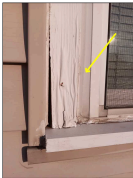
Peeling paint and wood deterioration to the exterior window frames and trim
