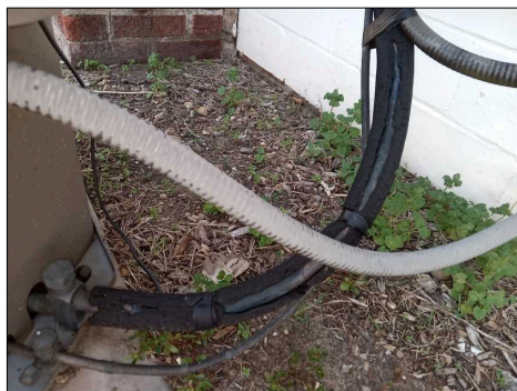
Deteriorated insulation on the a/c lines
