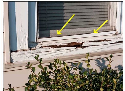
Peeling paint and wood deterioration to the exterior window frames and trim
