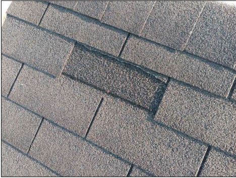
Broken/missing shingle tab
