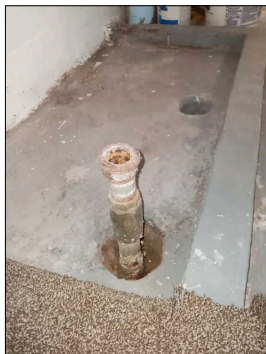
Old shallow well pipe should be capped
