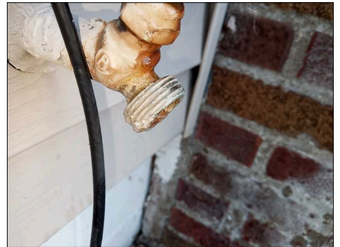
The north exterior hose bib has corroded hose threads
