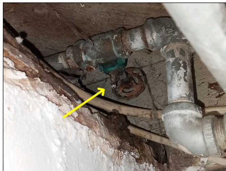
There is an active drip/leak in the plumbing visible from the basement
