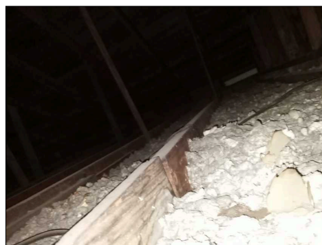
Insufficient attic space insulation
