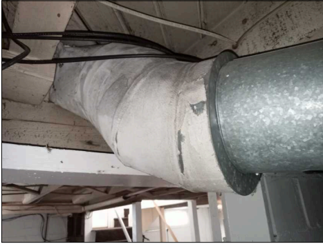
Fibertape on duct lines
