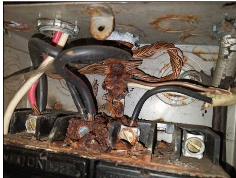
Extensive rusting and corrosion in a sub panel in the basement
