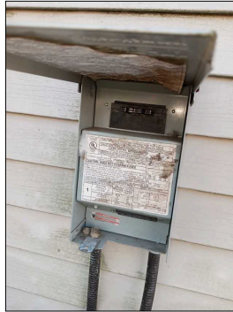
View of the a/c unit electrical disconnect
