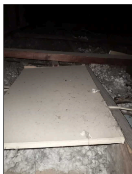
The access panel is not insulated
