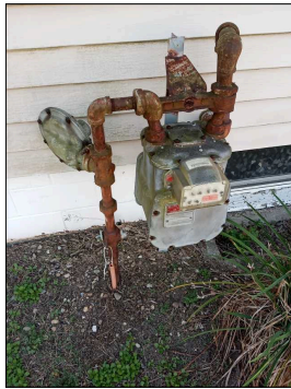
View of the gas meter and main shut off
