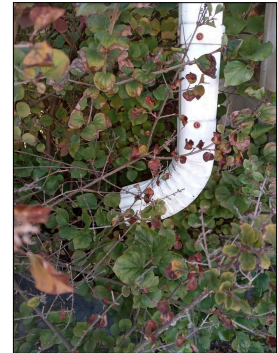
A downspout is missing an extension
