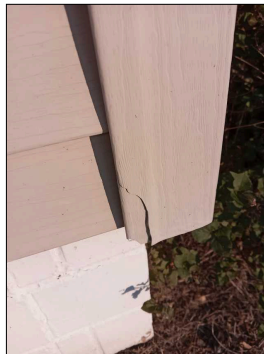
Cracked exterior siding
