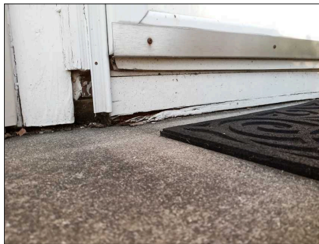
Peeling paint and wood deterioration to the exterior door frames and trim
