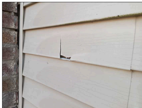
Hole in the exterior siding
