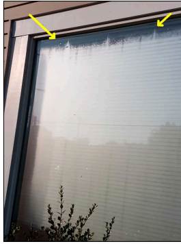
Moisture staining between the glass panes
