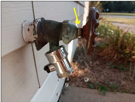
The south exterior hose bib leaks at the handle
