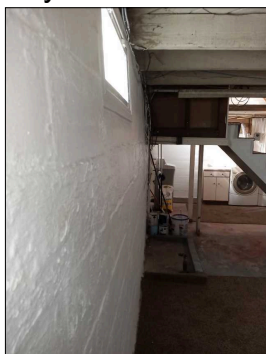
Bowing to the foundation
