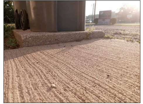
Unevenness to the sidewalk concrete possibly posing a trip hazard
