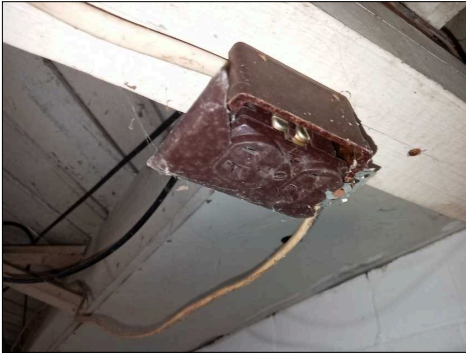
A basement outlet has a damaged cover plate
