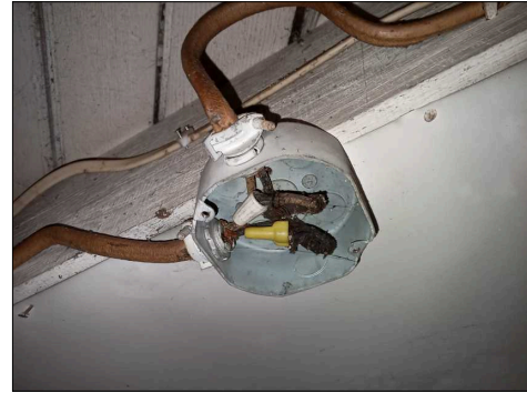
A basement junction box is missing a cover plate
