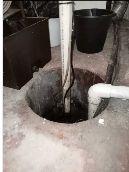
The sump pit cover is missing
