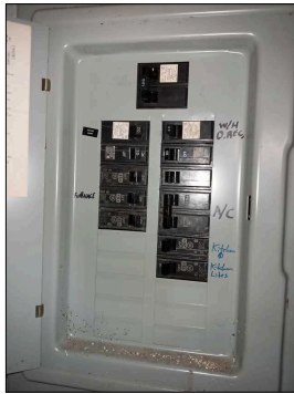
The electrical panel is not properly or completely labeled
