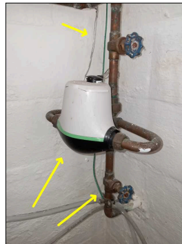
View of the main water shut off and meter
