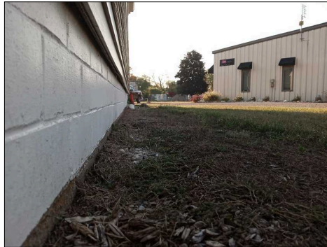
Flat to negative slope for drainage
