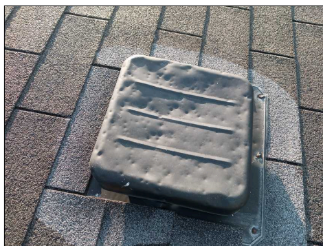
Dings or dents to the roof box vents
