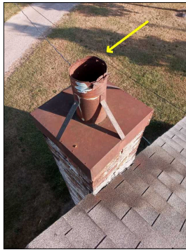
Missing metal screened flue pipe cover
