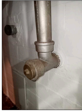
View of the main sewer clean out (interior)
