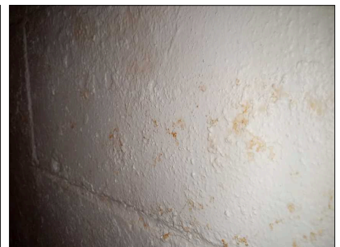
There is some moisture staining and scaling to the foundation visible from the basement
