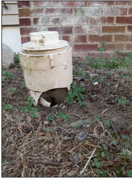
The north sewer clean out is damaged
